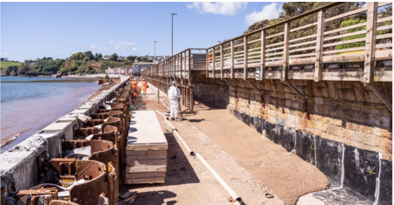
Ultra low-carbon concrete being placed at the Dawlish sea wall project
