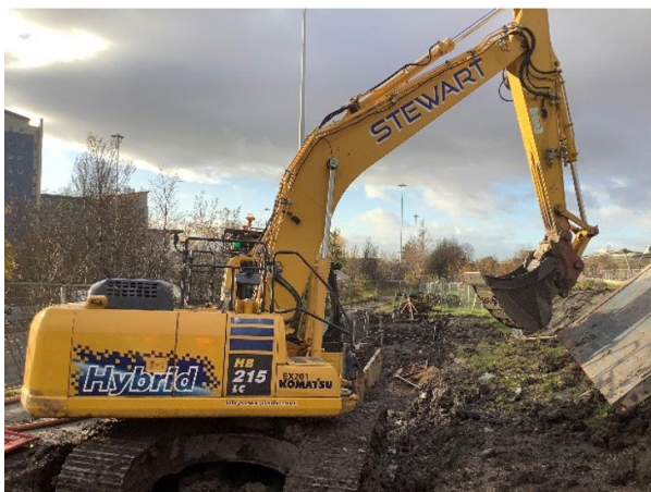
22t Hybrid excavator in action at the M8 footbridge scheme
